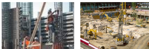
Figure 3. Construction site logistics
